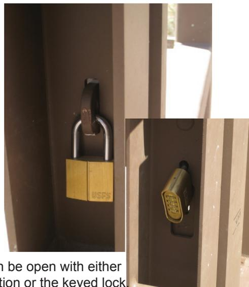
The gate can be open with either the combination or the keyed lock.
