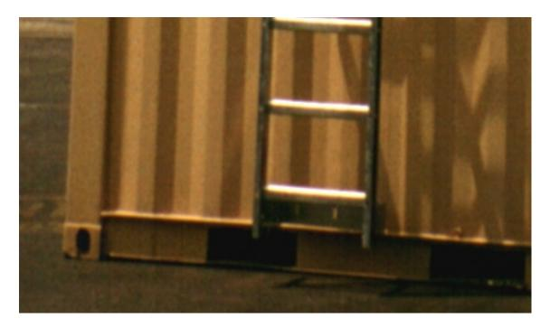
Bolt the bottom of the ladder in place to the container using two 5/16" bolts, four flat washers (one on each side of the assembly), and a pair of nuts. This will make the ladder more stable during use.
