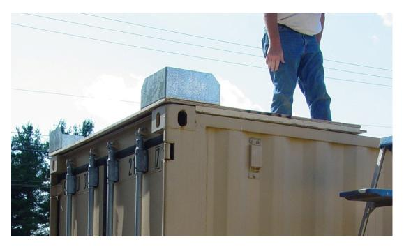
Position the rear floor panel such that it is snug and flush on the sides. Fasten the rear floor to the front floor panel down the seam using screws.
