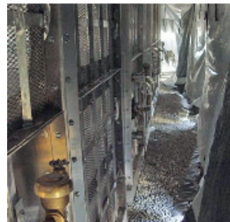
Rear view showing jail cells plumbed
