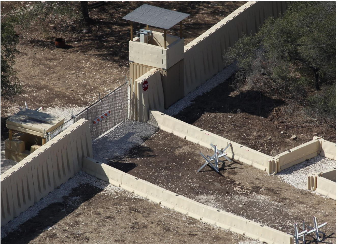
Photo shows a typical Entry Control set up. Bunker Checkpoint is on left side of photo.
