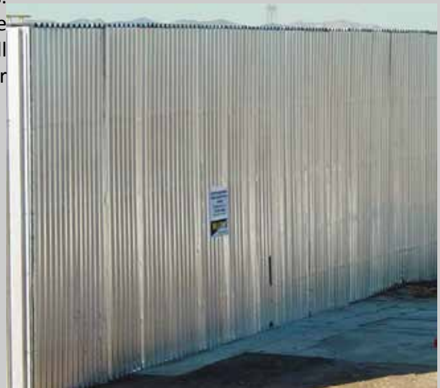
Completed 16' High Revetment Wall Section
