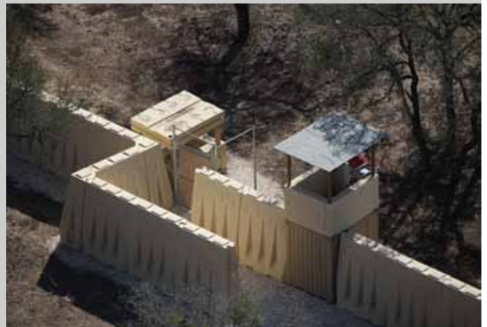
The Personnel Entry Control Point above includes: Houston Barricades, Bunker Check Point, Guard Tower and Man Gate.
